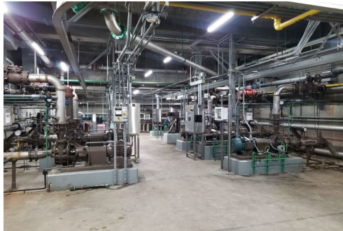
Photo: Primary Sludge Pump Station
