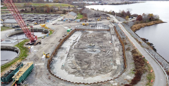
Photo: Construction Underway - Clarifiers at Bucklin Point
