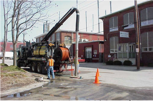
Photo: Interceptor Grit Removal
