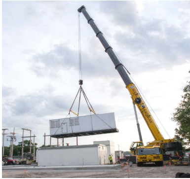
Photo: 2,000 kWh Generator Installation
