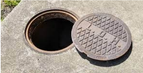
Photo: Municipal Sewer Manhole Cover
