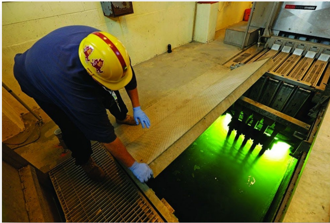
Bucklin Point UV Disinfection System
