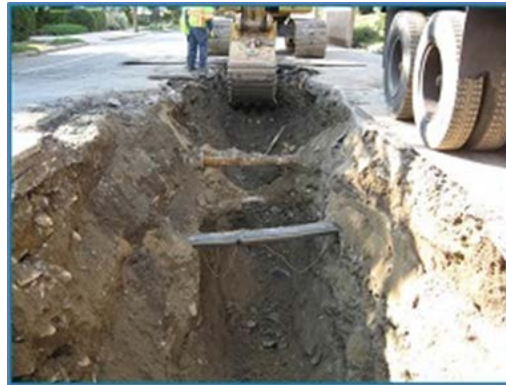
Figure 19 - NBC Phase II Sewer Separation Utility Conflicts
