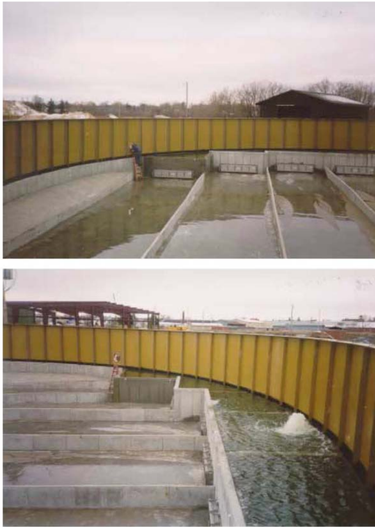
Figure 56 – Circular CSO Storage Tank with Flush Gates
