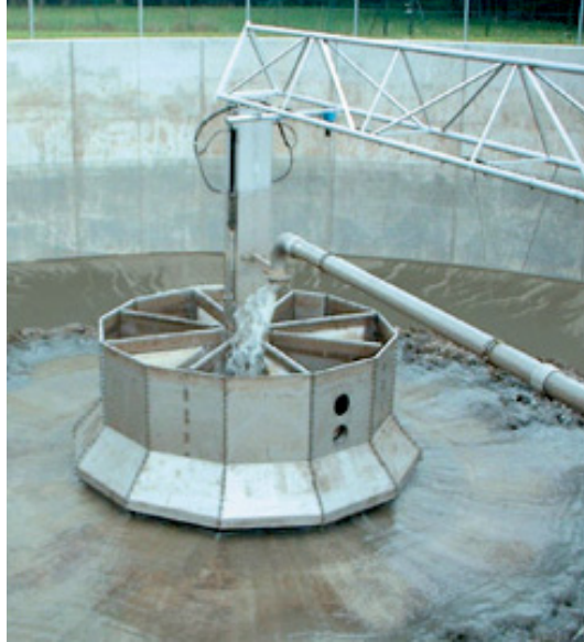
Figure 57 – Example of Round Tank Flushing System
