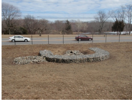
Figure 4 - Stormwater Flow Control - Detention Storage
