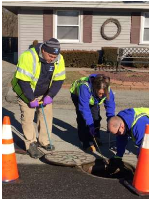
Environmental monitors conducting sanitary manhole sampling
