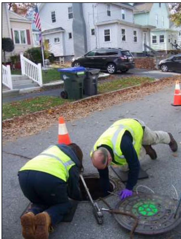
Environmental monitors conducting sanitary manhole sampling
