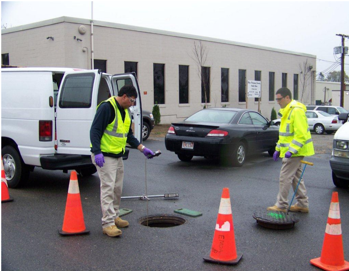
NBC EMDA staff Installing an Industrial Manhole Sampler
